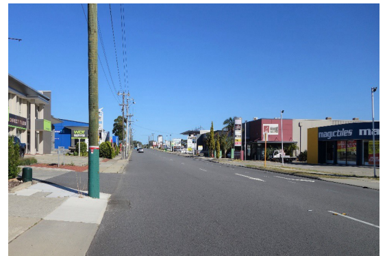
Image 2: Example Road Environment – Industrial Area
