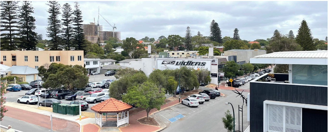
Figure 15: Site Images of the Cottesloe Town Centre
