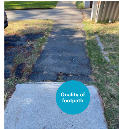
At some points major defects have more than 15mm level difference, creating a potential trip hazard and difficulty navigating in a wheel chair or pushing a pram
