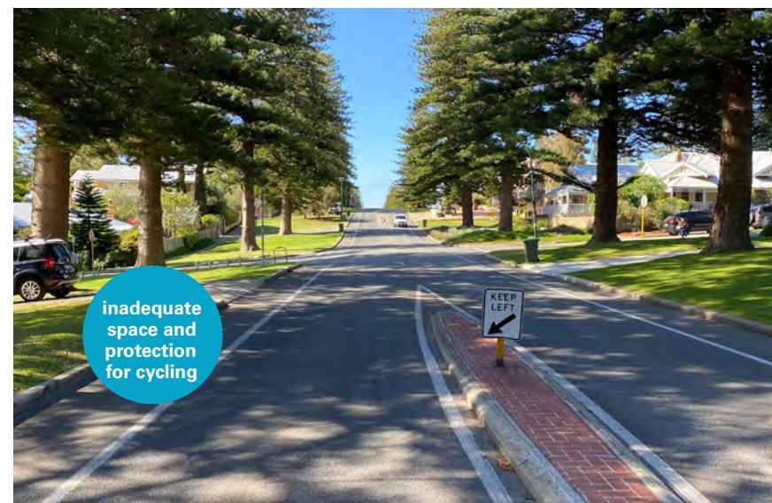
Painted white line shoulders are not sufficient protection for people cycling given traffic speeds of 50km/h. Shared space for cycling appropriate at 30km/h.
