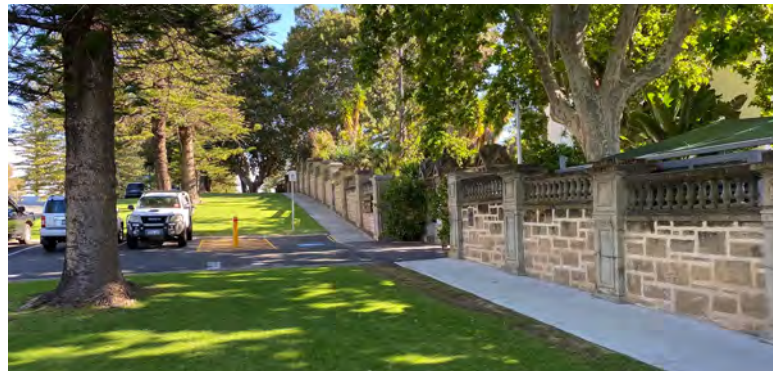
Masonry street walls define street edge adjacent Cottesloe Civic Centre
