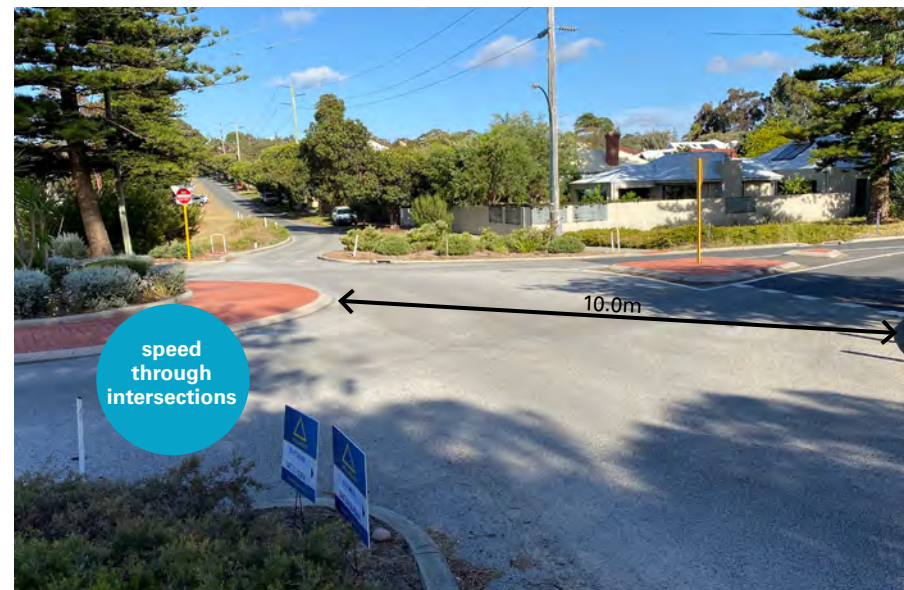
Road pavement on Grant Street roundabouts is very large encouraging vehicles to travel at dangerous speeds through the intersection.
