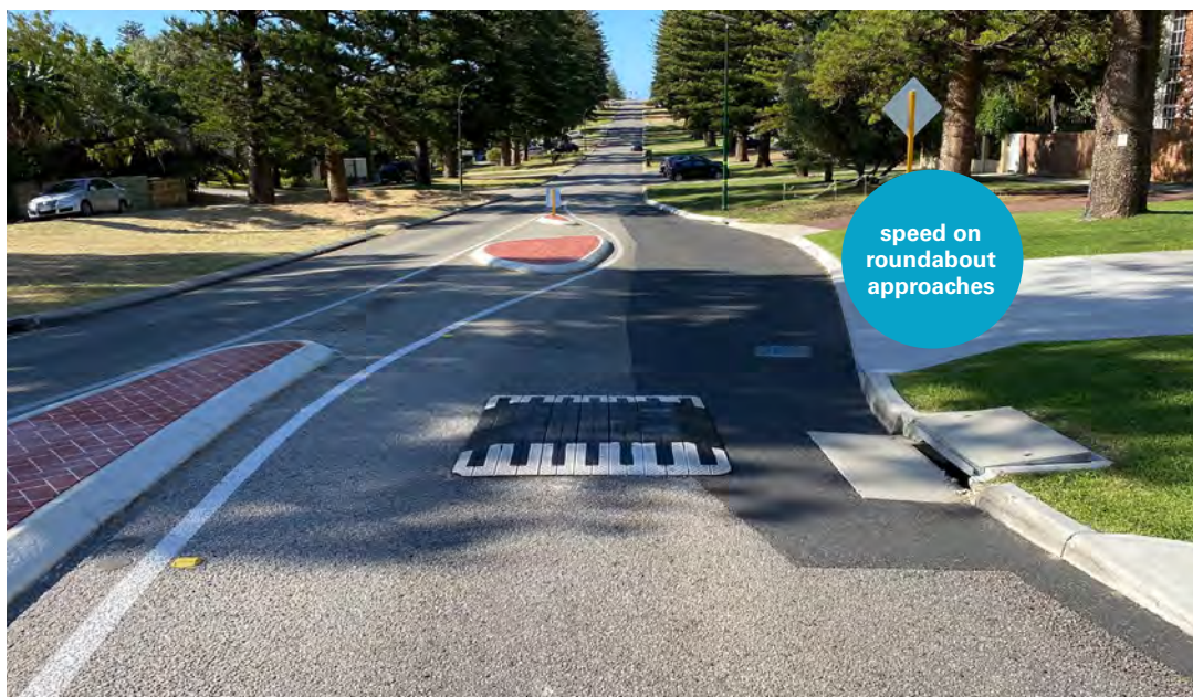
Road pavement approaches to roundabouts designed with generous swept paths for larger vehicles meaning most vehicles are still carrying speed entering roundabouts. No priority for people walking.
